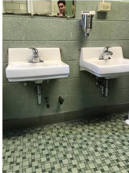
Second Floor Lavatories
