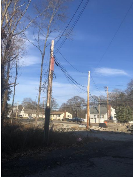
Existing Utility Pole
